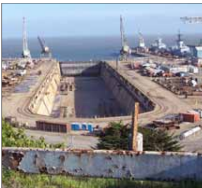
The dry-docks on the Shipyard
